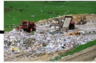
Existing Landfill Excavated to remove historic MSW
